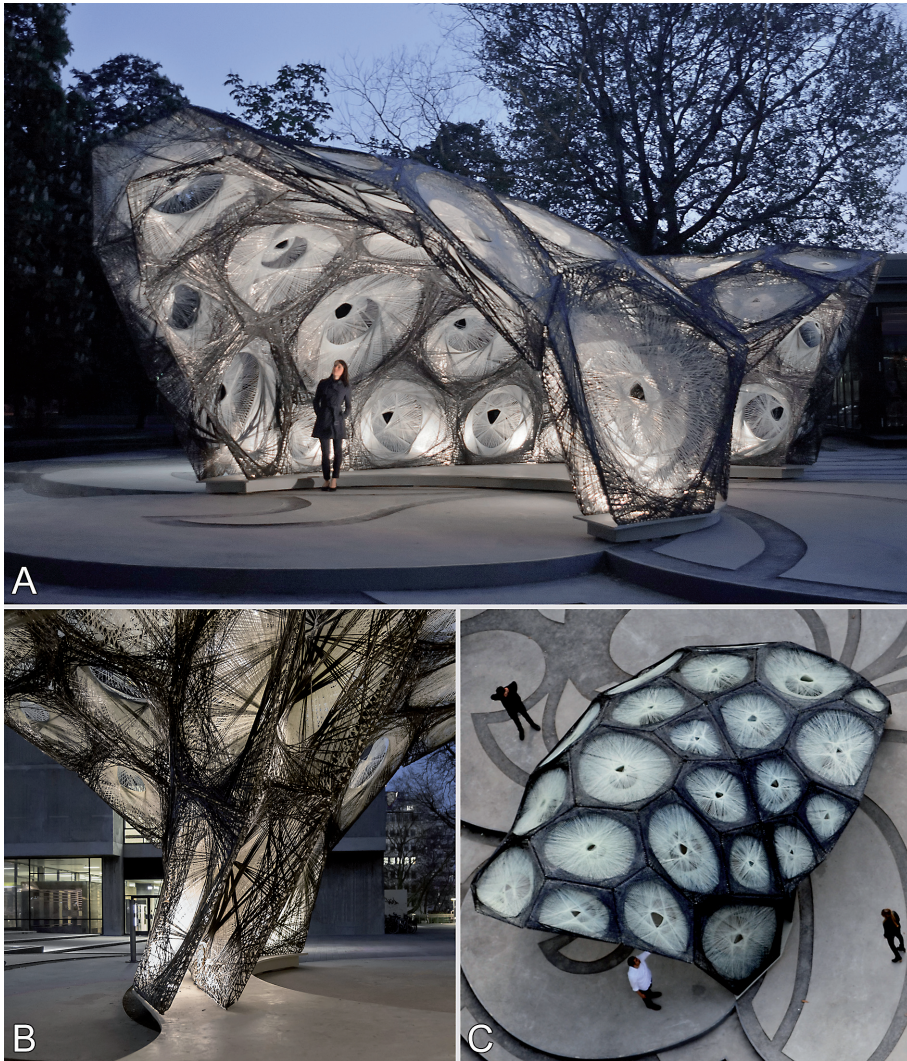
Fig. 3: Completed research pavilion at the campus of the University of Stuttgart. A Front view. B View from inside; note the fiber construction and the two walls. C Top view.
